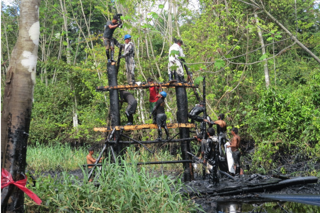
Photo 3: Cuninico residents inserting removing one of the wooden timber frames the supports the North Peruvian pipeline. The absence of heavy lifting equipment and limited white protective overalls are clearly visible (Photo given to me by a Cuninico resident who himself received it from a Petroperu worker and used with their permission, June 2014).
